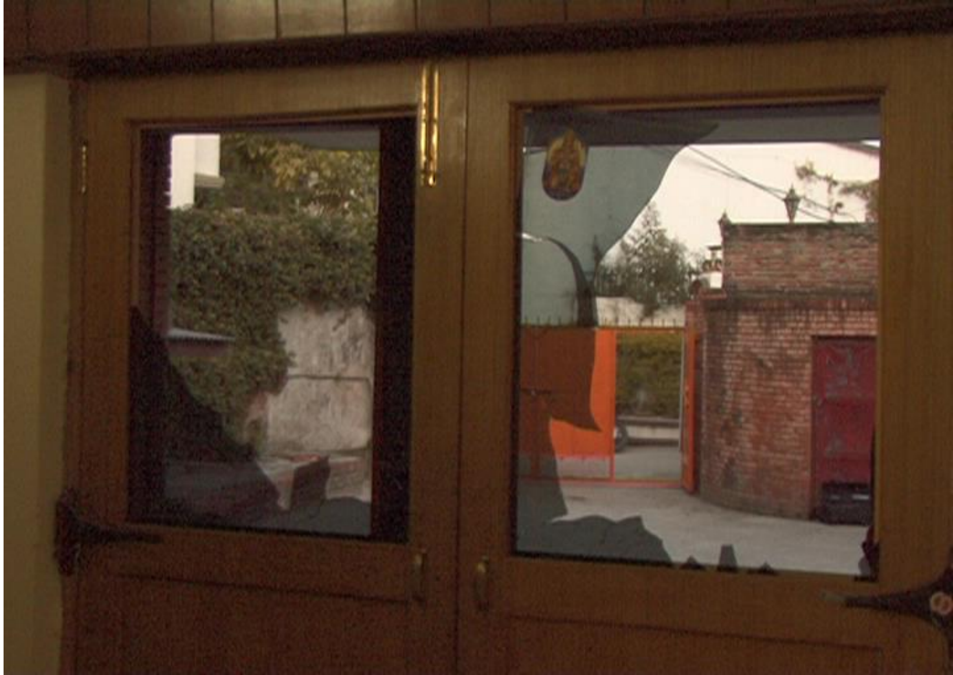
Picture 2. Damaged Infrastructure of health set-up by perpetrators
